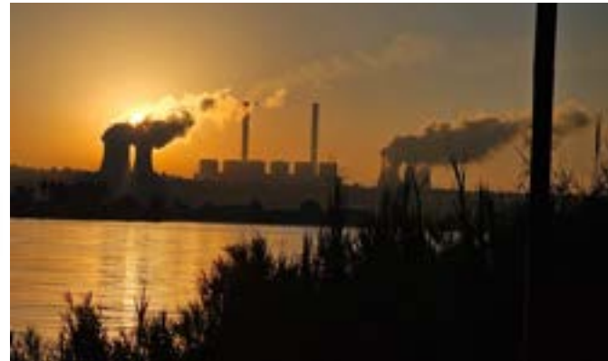
Duvha Power Station near Bezrus
